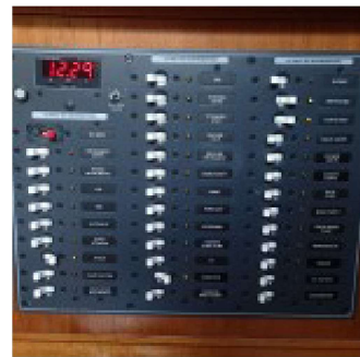
DC distribution board
