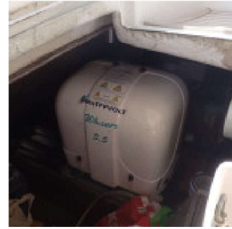
Silent diesel generator
